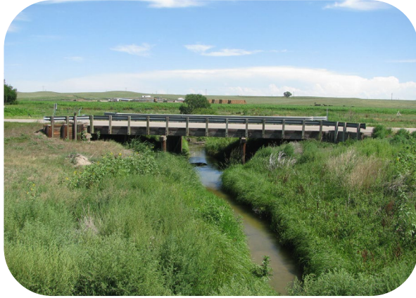
US 6 over UPRR; Platte River; Beaver Canal in Morgan County (C-22-K)
