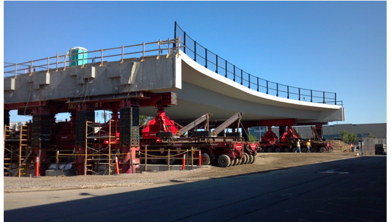
Accelerated Bridge Construction using SPMT (Pecos over I-70 - E-16-YQ)
