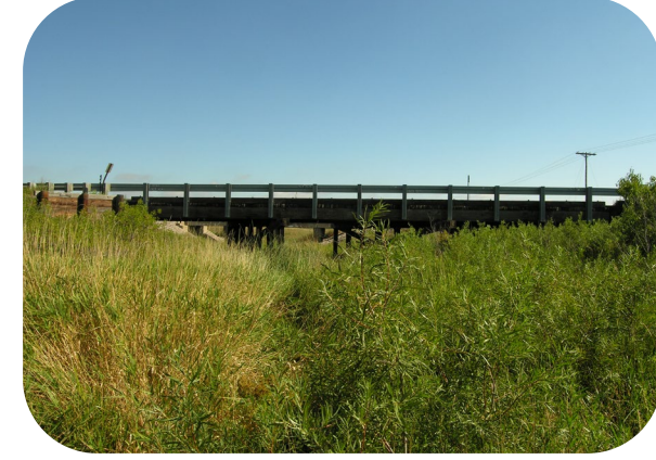
US 34 over Republican River in Yuma County (D-28-D)
