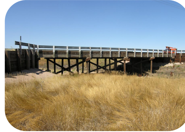
SH 61 over Surveyor Creek in Washington County (D-25-E)
